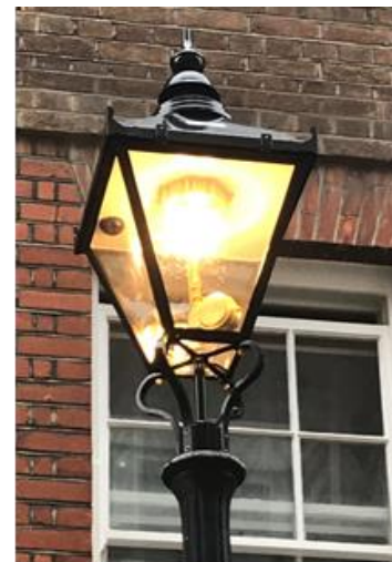
2 nd generation gas mimic lantern installed in Queen Anne's Gate and Abbey Orchard Street
