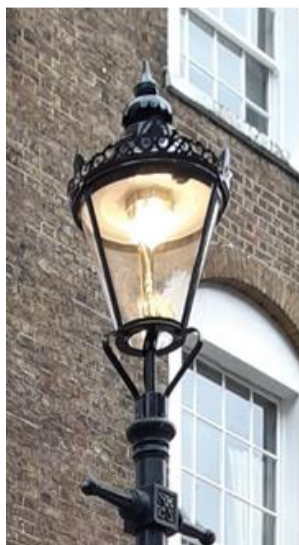
2 nd generation gas mimic lantern installed in Queen Anne's Gate and Abbey Orchard Street
